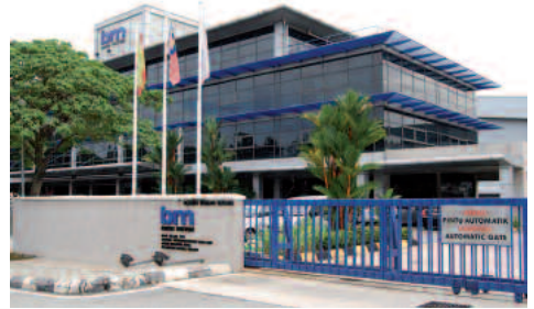
Office in Kuala Lumpur and warehouse next door
